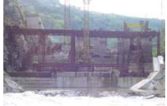
Huge projects require large amounts of timber for adequate housing infrastructure
